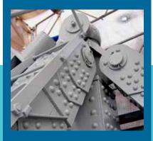
Our oil alkyd system is ideal for complex constructions like riveted bridges, cranes with lots of crevices or where surface tolerance is the main concern.
